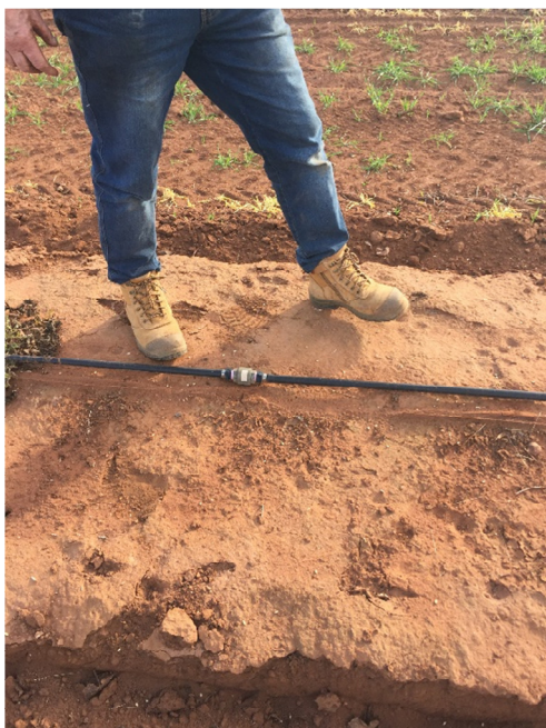
Figure 1. Dripline non leakage valve installed on a lateral
